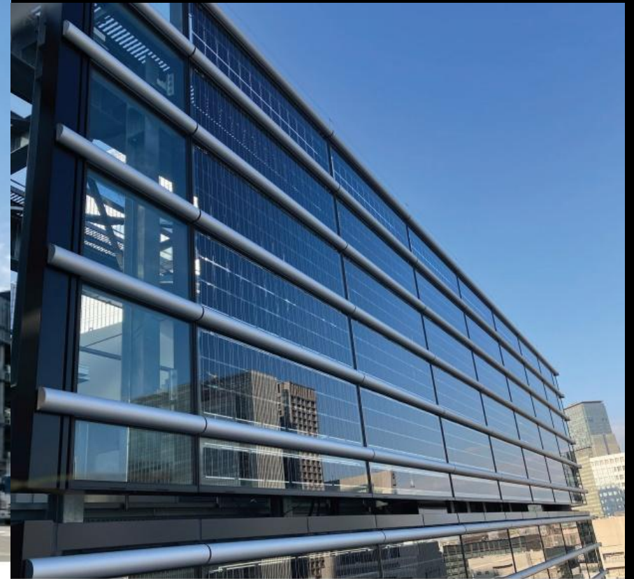
Close-up detail of the BIPV curtain wall.
